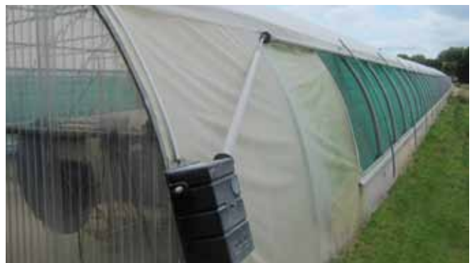
Films opened by cable and mechanised winch
